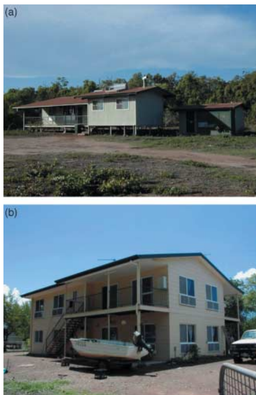
Figure 6 Change in house design standard for two large families from 1995 (top) to 2000 (bottom).
